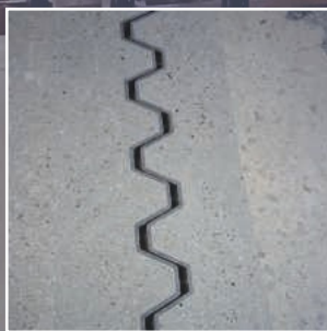
Permaneo joint repairs
